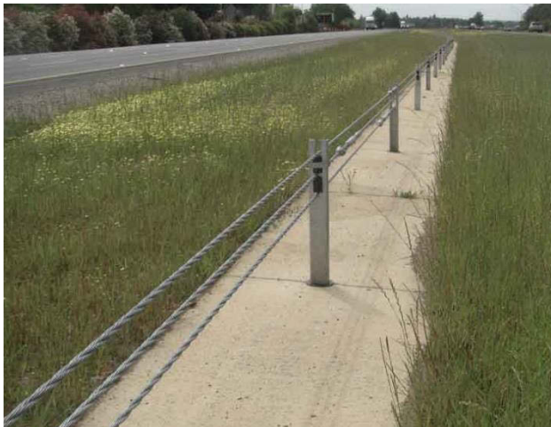
A cable barrier is less costly than metal beam guardrail and can be easier to maintain.
