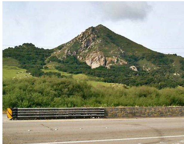
Type 60 Textured concrete barrier along Highway 1, San Luis Obispo, CA. (Source: District 5 Landscape Architecture Office)
