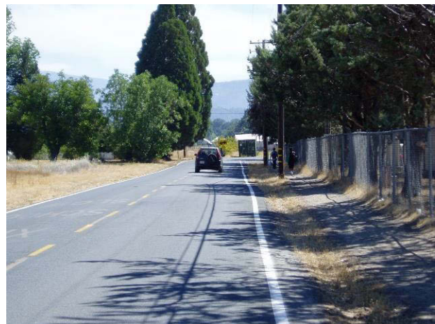
Figure 164: Foothill Blvd. at school looking east
