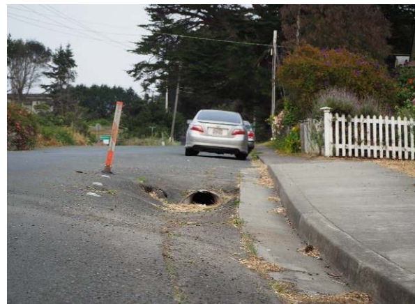
Figure 3: Open drainage along Riverside Drive
