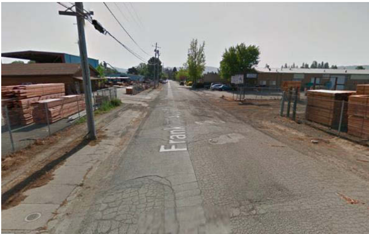
Figure 123: Franklin Street, looking east from Blosser lane (Source: Google Street View)
