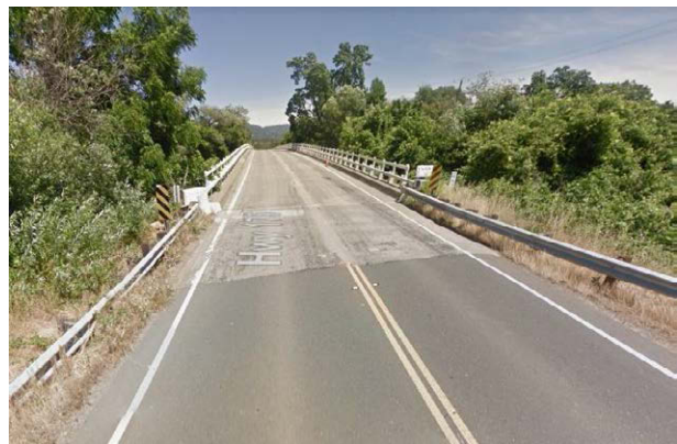
Figure 178: Russian River Bridge on Highway 175, looking east (Source: Google Street View)
