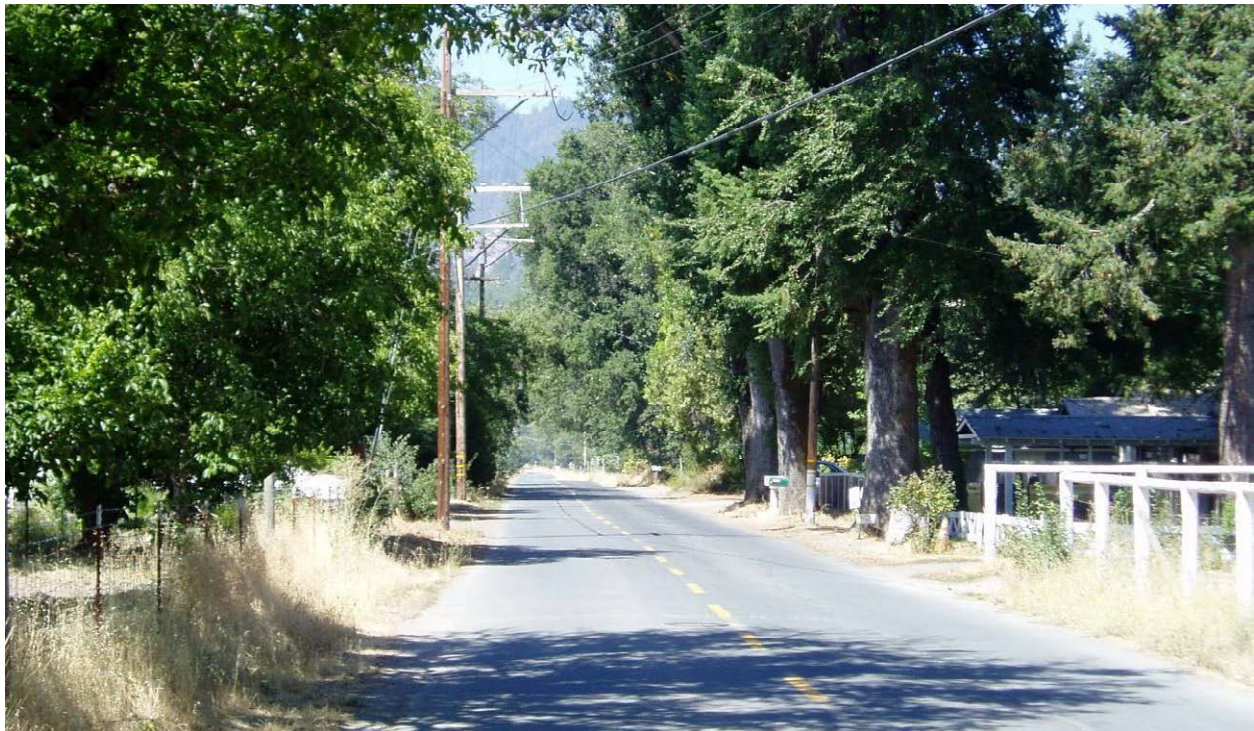
Figure 165: Highway 162 north of Covelo looking north
