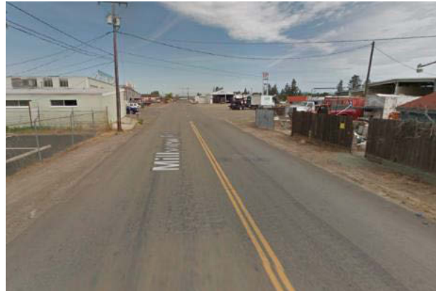
Figure 102: Missing sidewalks on Millview Road (Source: Google Street View)
