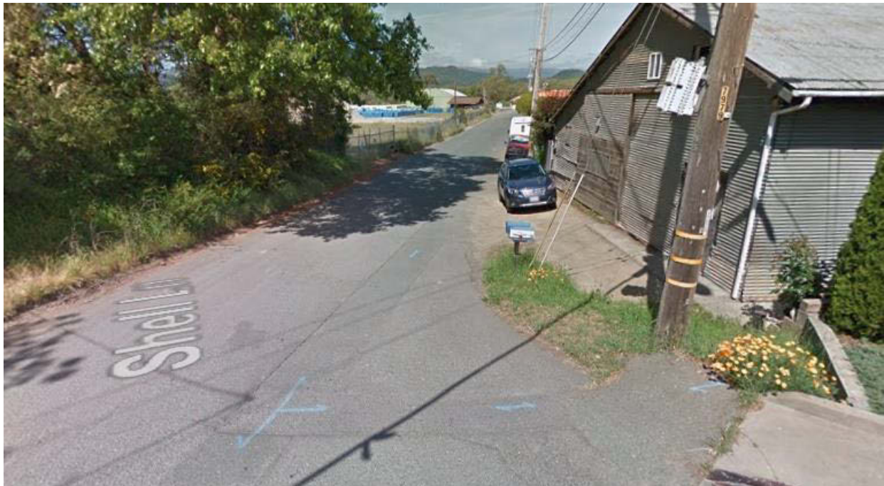
Figure 130: Shell Lane has an identified need for sidewalks and curb ramps at the intersection with Baechtel Road (Source: Google Street View)
