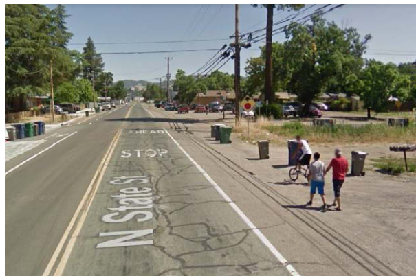
Figure 158: Looking North on State Street and Hopkins Street intersection in Calpella (Source: Google Street View)
