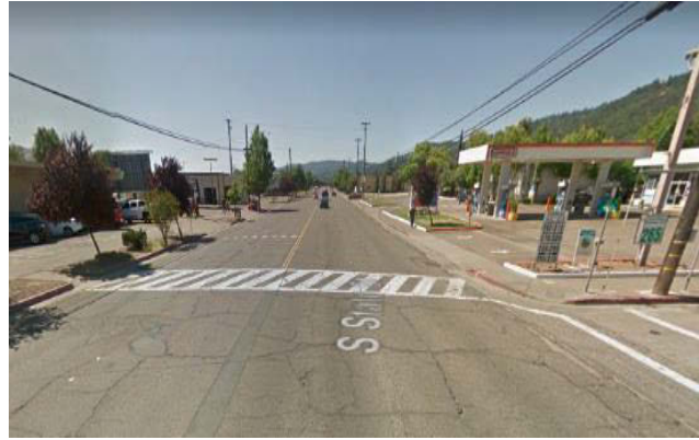
Figure 87: Intersection of Luce Avenue and North State Street, looking south (Source: Google Street View)
