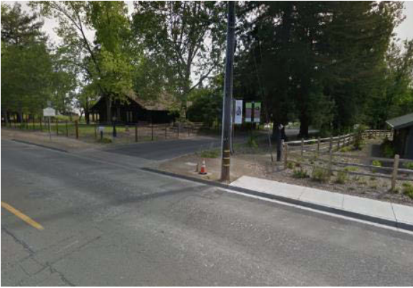
Figure 68: Main Street, between Clay and Cleveland Street with sidewalk missing (Source: Google Street View)
