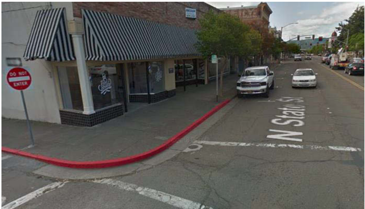
Figure 97: The intersection of North State Street and Smith Street lacks ADA accessible curb ramps (Source: Google Street View)
