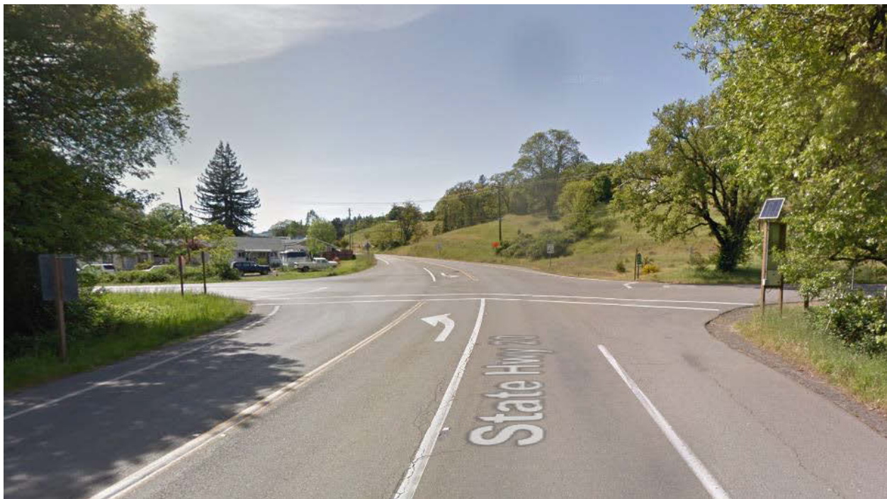
Figure 125: Intersection of Highway 20 and Blosser Lane, looking west
