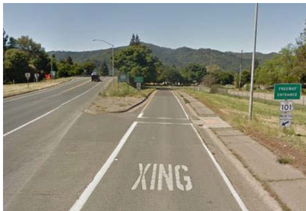
Figure 106: Talmage Road and US Highway 101 Interchange, Looking West (Source: Google Street View)
