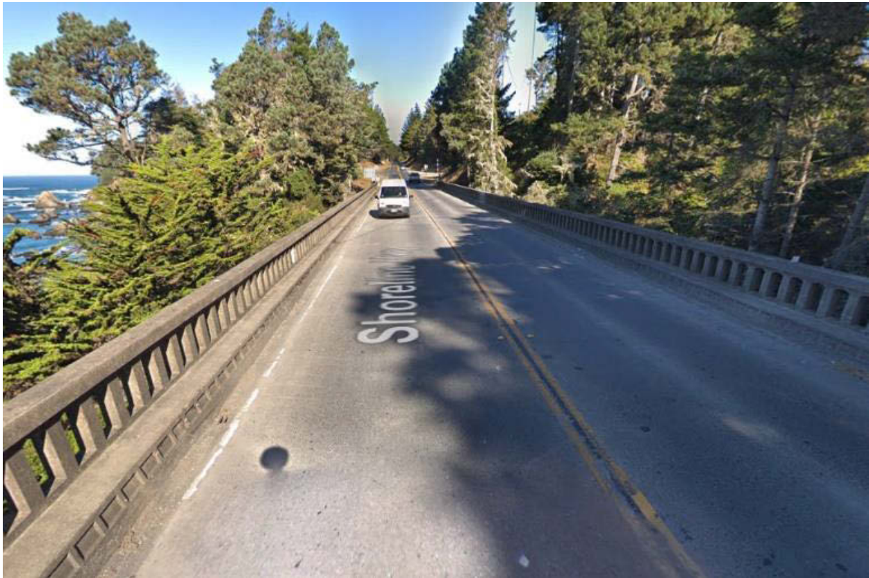
Figure 191: Jack Peters Creek Bridge features narrow shoulders and is inaccessible for pedestrians. (Source: Google Street View)
