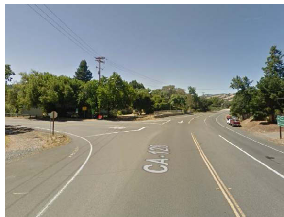
Figure 147: Highway 128 and Mountain View Road Intersection, near Anderson Valley Jr./Sr. High School (Source: Google Street view)
