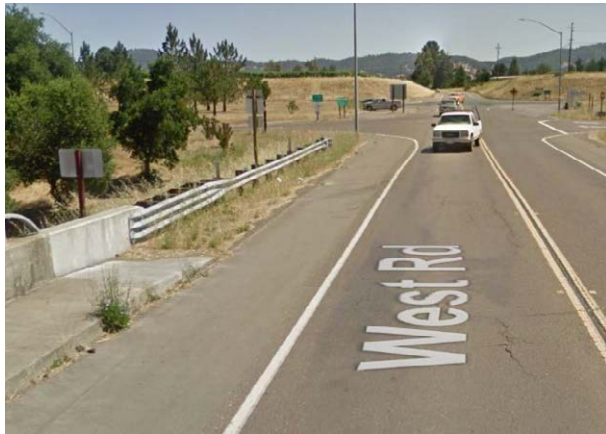
Figure 201: End of Sidewalk on West Road Bridge, looking north (Source: Google Street View)
