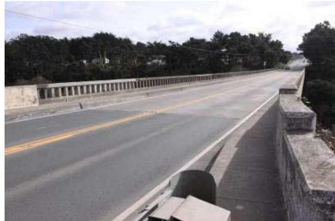
Figure 48: Hare Creel Bridge western sidewalk
