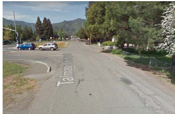
Figure 89: Talmage Frontage Road near Loraine Street (Source: Google Street View)
