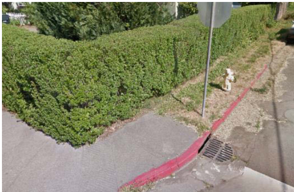
Figure 116: The Intersection of North Street and Pine Street is missing sidewalks (Source: Google Street View)
