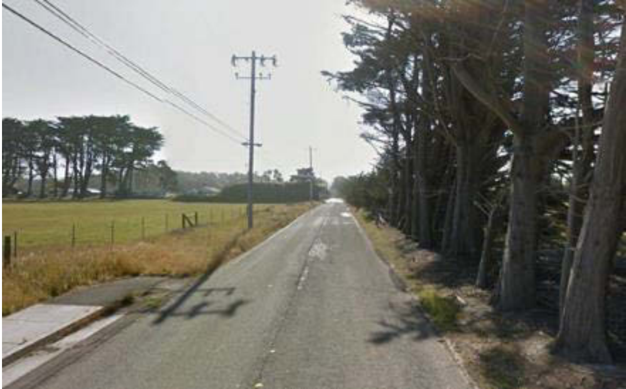
Figure 46: Airport Road, looking east (Source: Google Street View)
