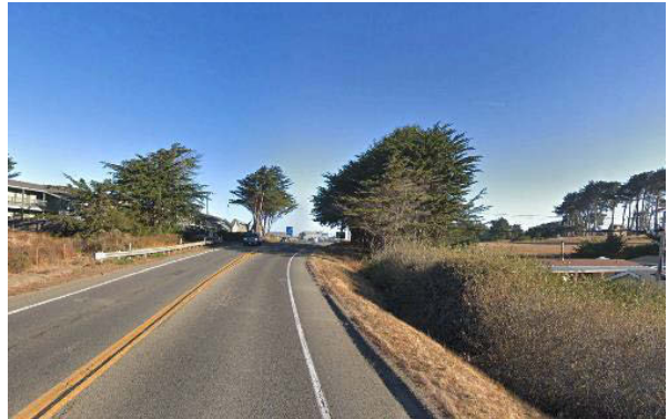
Figure 28: Narrow shoulder on Highway 1 between Airport Road and Pudding Creek Road (Source: Google Street View)
