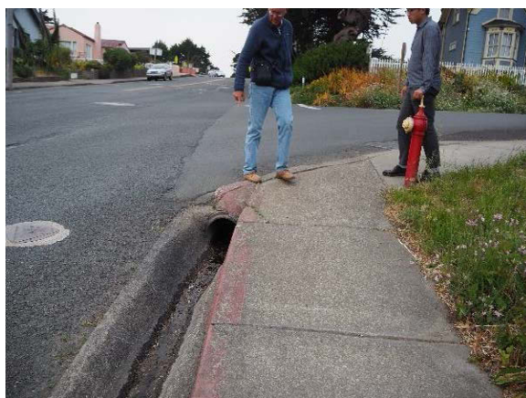
Figure 4: Open drainage along Main St./Hwy 1
