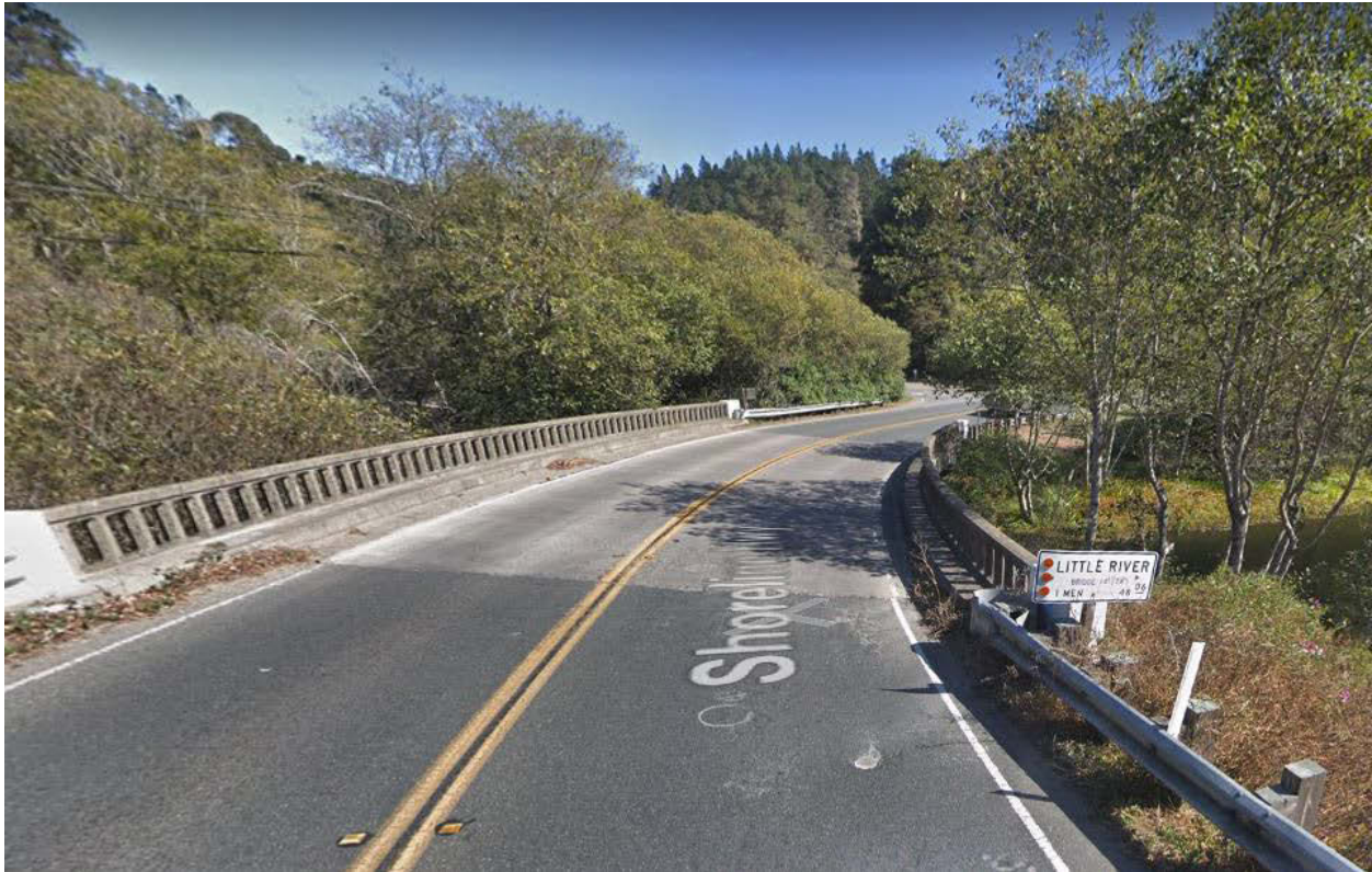
Figure 190: Little River Bridge, looking south (Source: Google Street View)
