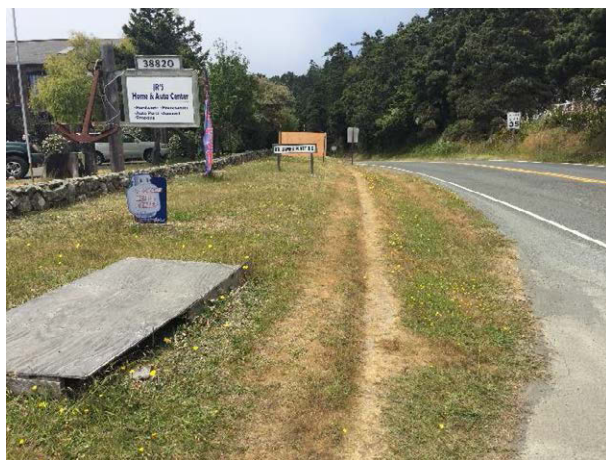
Figure 18: Informal Path on west side
