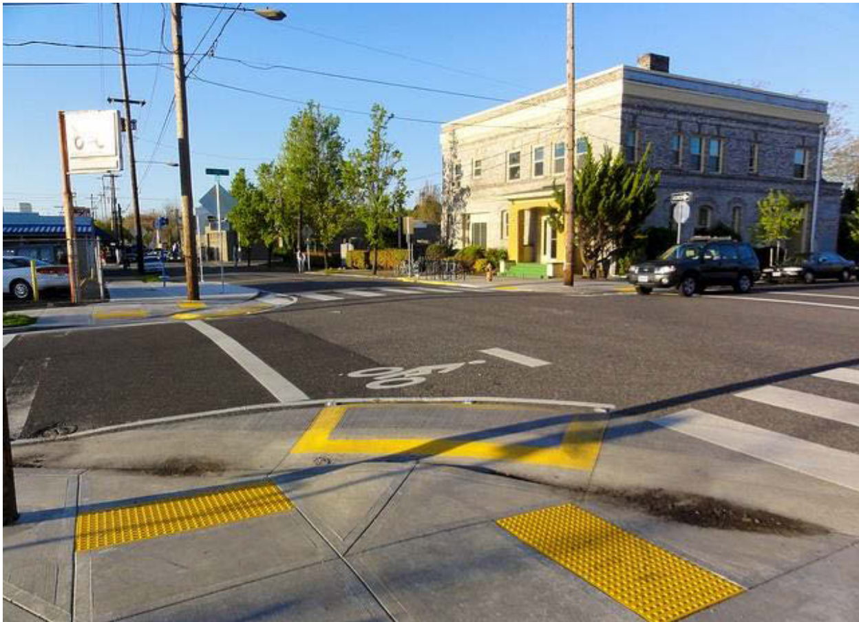
Figure 108: Mountable curb (Source: Google Images)
