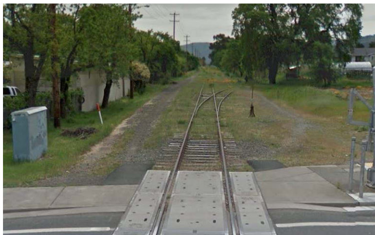
Figure 91: North Western Railway line, looking south from East Gobbi Street (Source: Google Street View)
