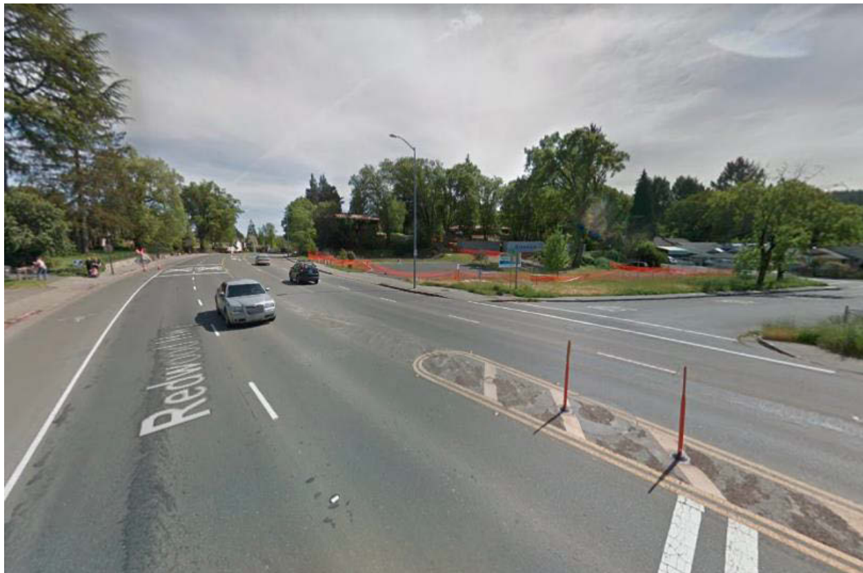
Figure 126: The intersection of Walnut Street and South Main Street does not have crossing facilities (Source: Google Street View)
