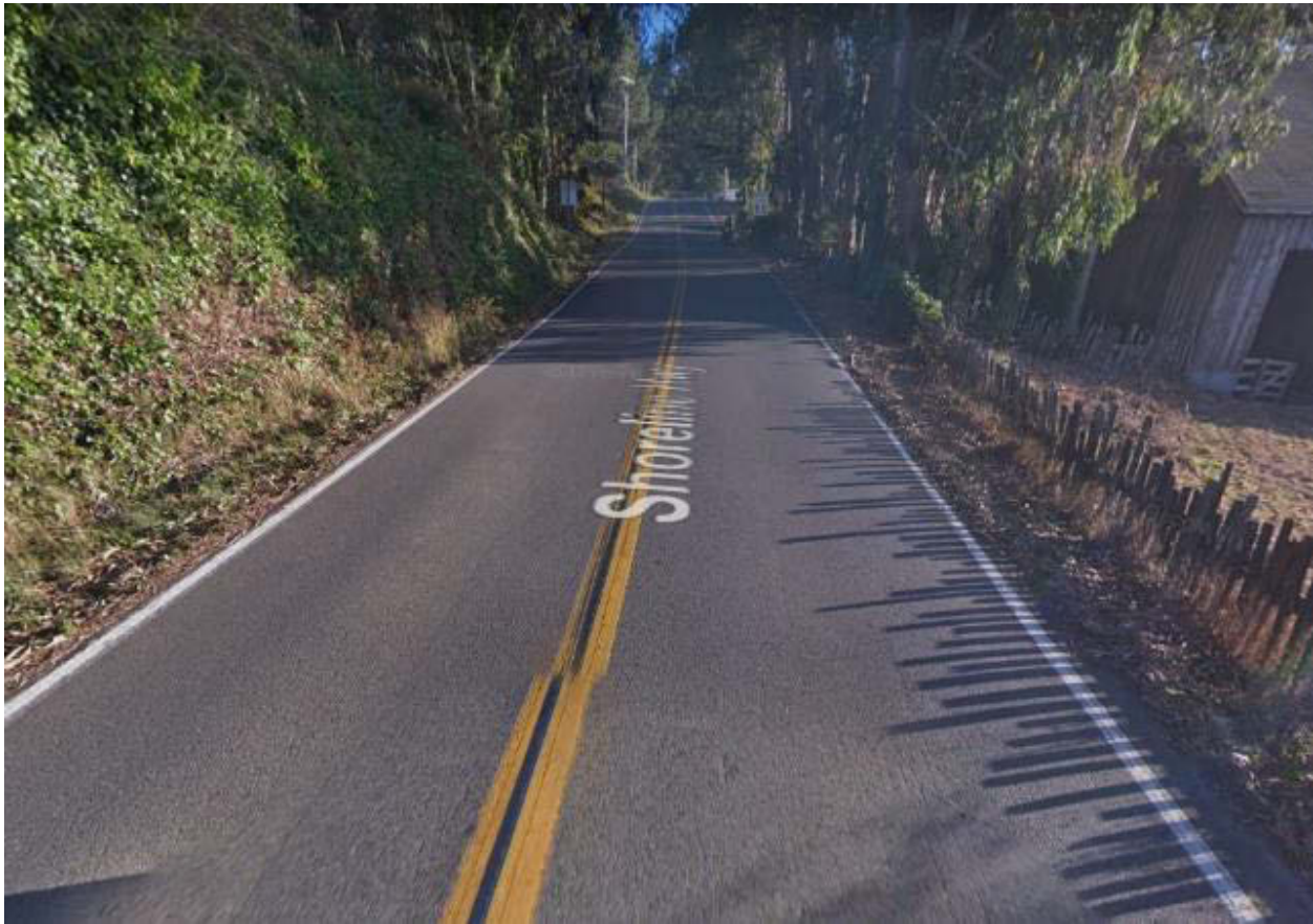
Figure 204: Highway 1 Features Narrow Shoulders South of Westport (Source: Google Street View)
