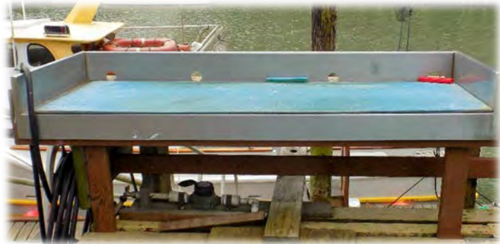
Existing North Side Fish Cleaning Station
