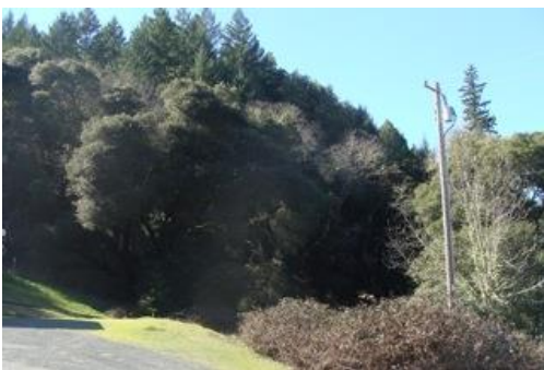
Utility pole drop for Yorkville Fire Station
