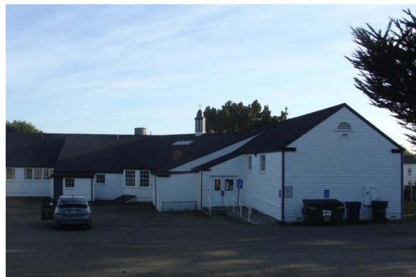
Parking lot to the north of the Community Center
