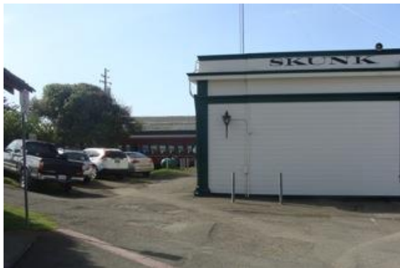
Utility drop on corner of building close to parking
