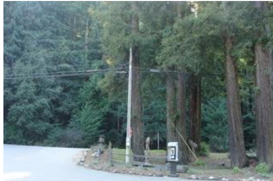
Utility pole adjacent to parking lot
