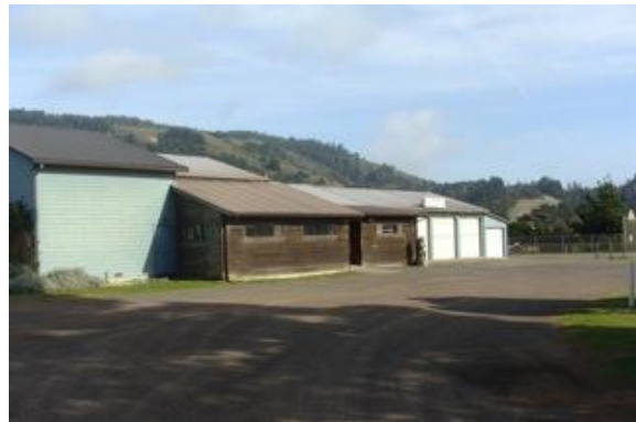
Gravel parking lot west of Community Center
