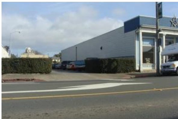
City Lot to the north of the PG&E building
