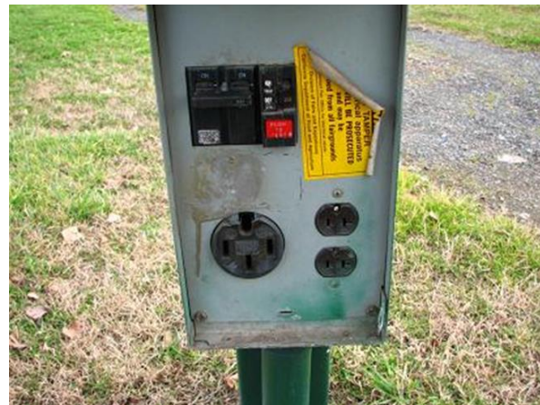
RV Park is on the southeast part of the fairgrounds. RV Pedestal with NEMA receptacle
