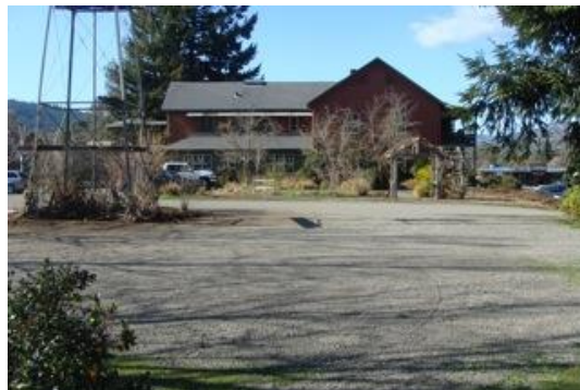
Boonville Hotel off-street parking
