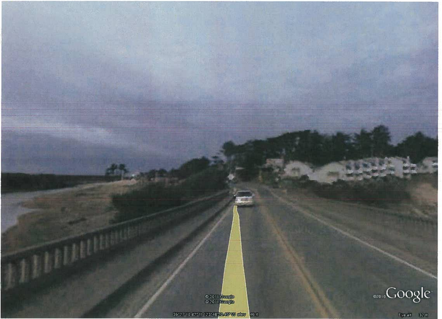
Pudding Creek Bridge
