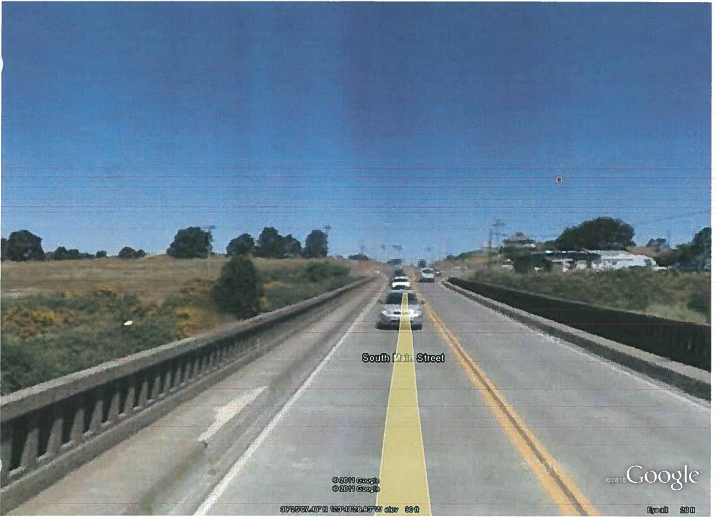
Hare Creek Bridge
