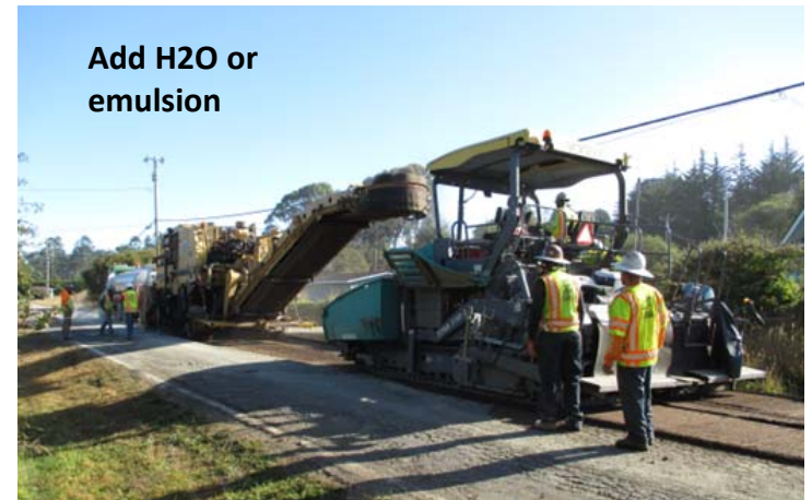
Compacted recycled AB w/ emulsion cement mix
