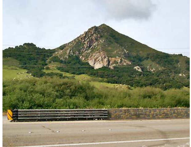
Type 60 Textured concrete barrier along Highway 1, San Luis Obispo, CA. (Photo credit: District 5 Landscape Architecture Office)
