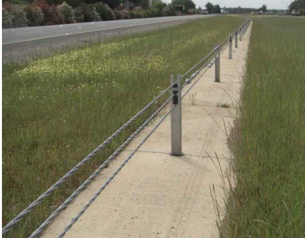
A cable barrier is less costly than metal beam guardrail and is can be easier to maintain.
